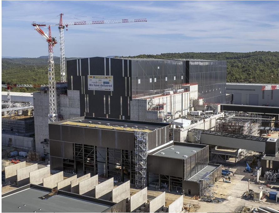
Iter machine hall, 9/2023
