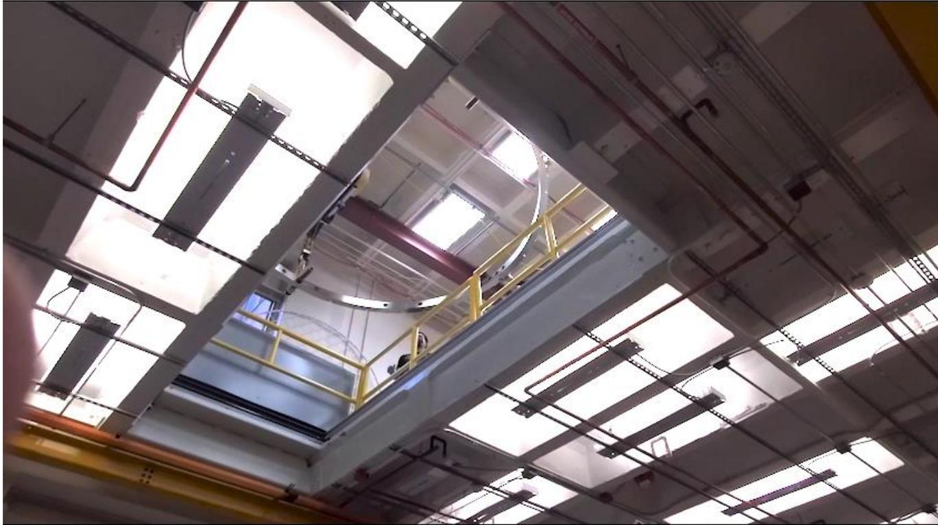
New insert provides improved diagnostic access, as well as quick turn-around between experimental configurations
