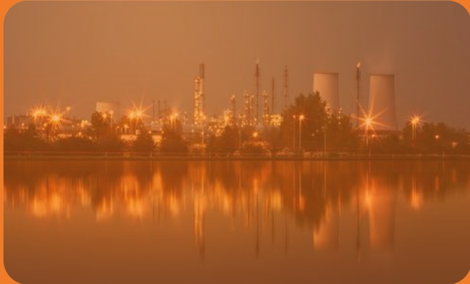
Fuel-based power plant: 13 Acres / MW
